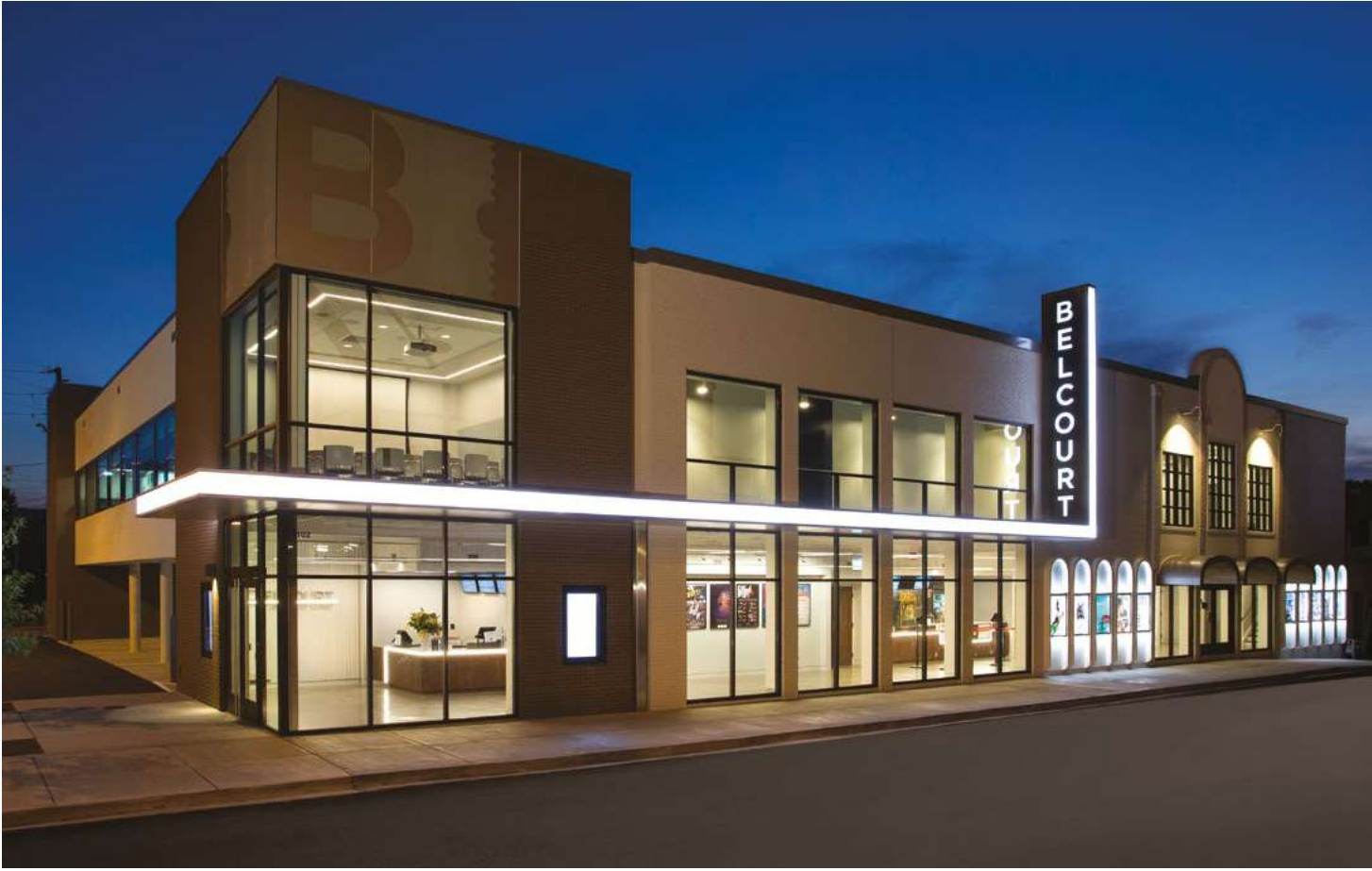
THE BELCOURT THEATRE, NASHVILLE, TENNESSEE, Architect: TUCK-HINTON ARCHITECTS PLC
